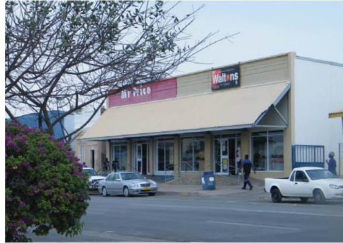
FIGURE 51: NEWER BUILDINGS WITH SHADE STRUCTURES
